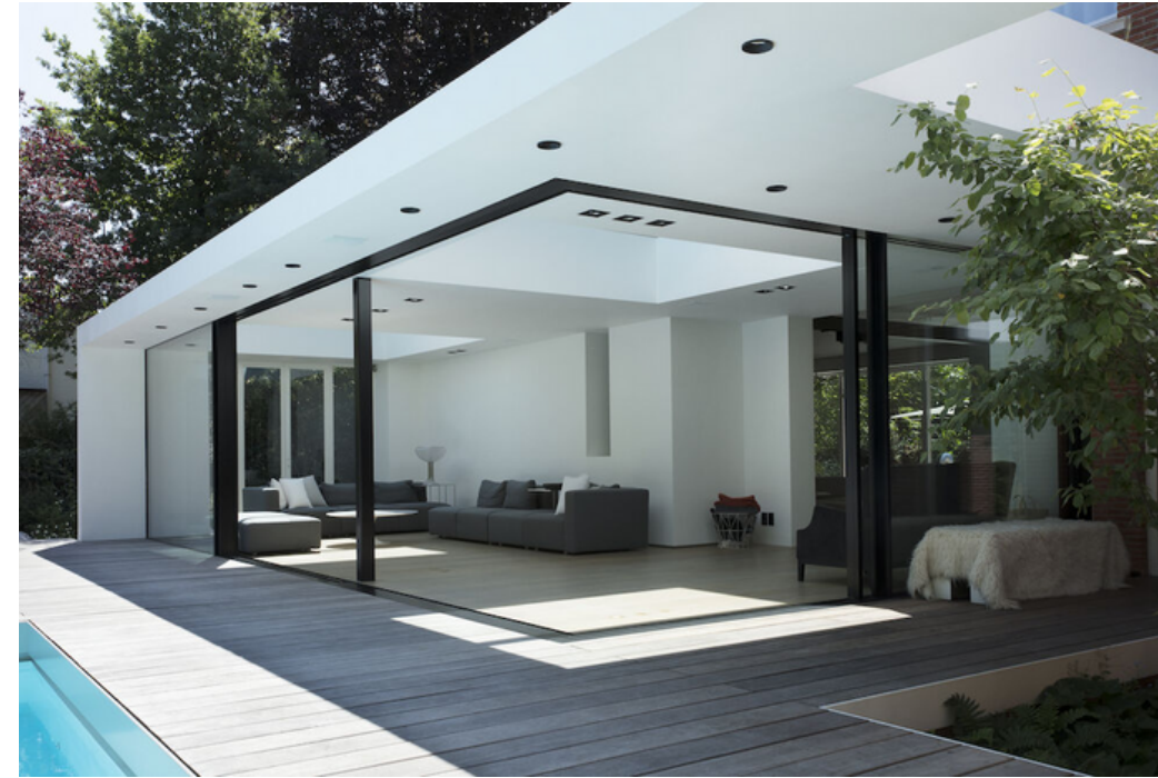
Project showing solution with opening corner
